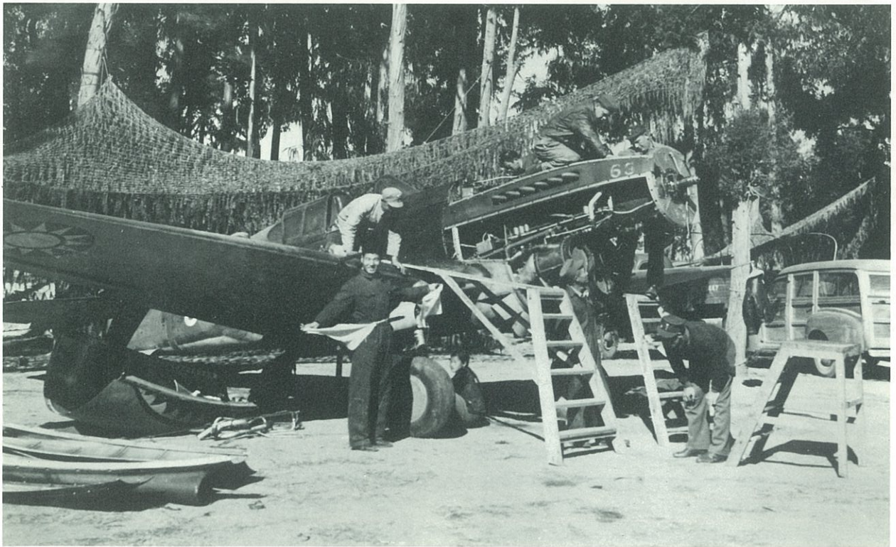
AVG'S AIR-CONDITIONED MAINTENANCE HANGAR
